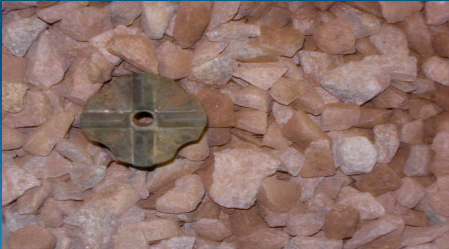
Fig 2.0 showing the Stemming Material (Chipping)
